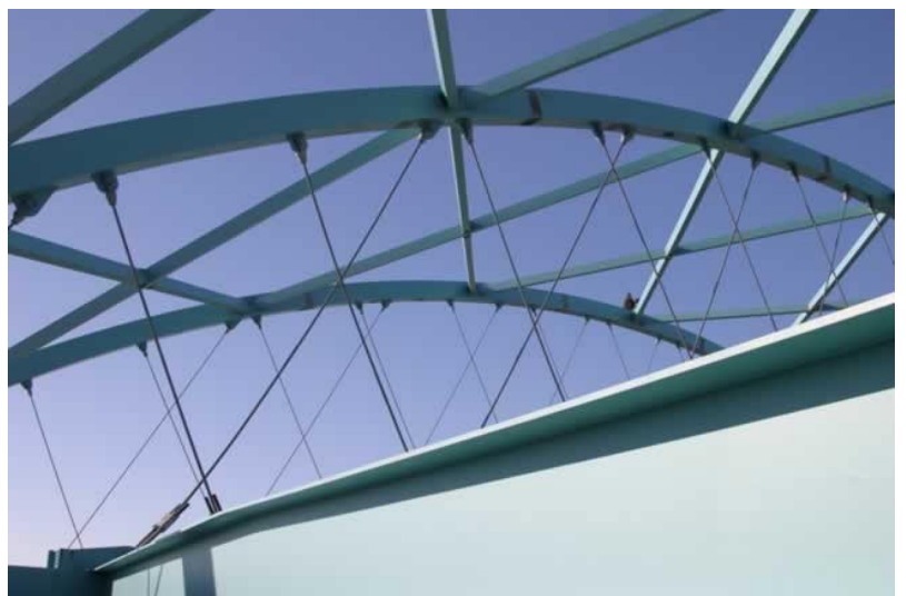
PHOTO 2: I-195 Relocation Bridge (Steel, 2006). Providence. Photo by RIDOT staff.
